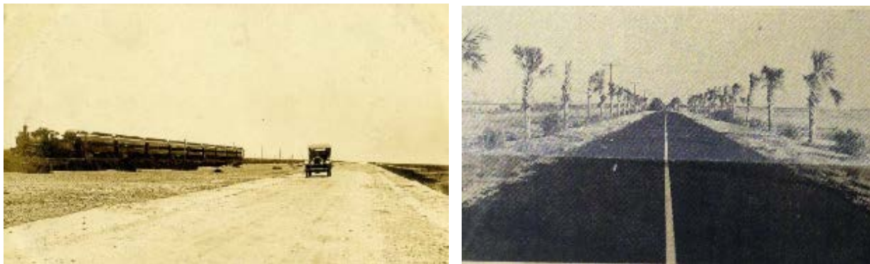
Figure 8. (Left) Unknown, The Road to Tybee Showing Constructed , 1923, Vertical File, Savannah Public Library, Savannah, GA. (Right) Unknown, Tybee Road, 14 Miles from Savannah & 40 Feet Wide. , 1924, Vertical File, Savannah Public Library, Savannah, GA.
